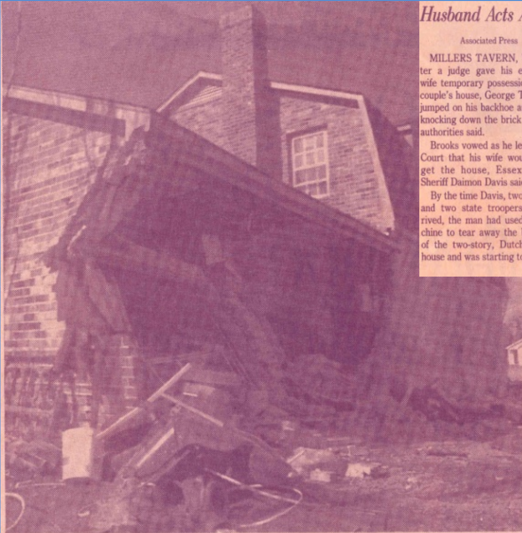
George T. Brooks reportedly used a backhoe to knock down the back wall of his two-story, Dutch colonial house.
